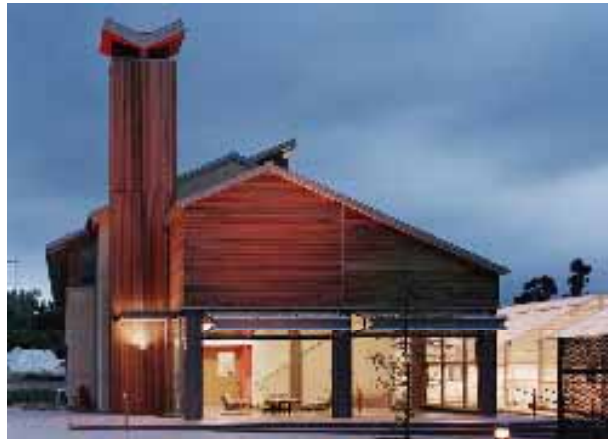
Figure 4.1 Global Ecology Research Center - Steel Frame
