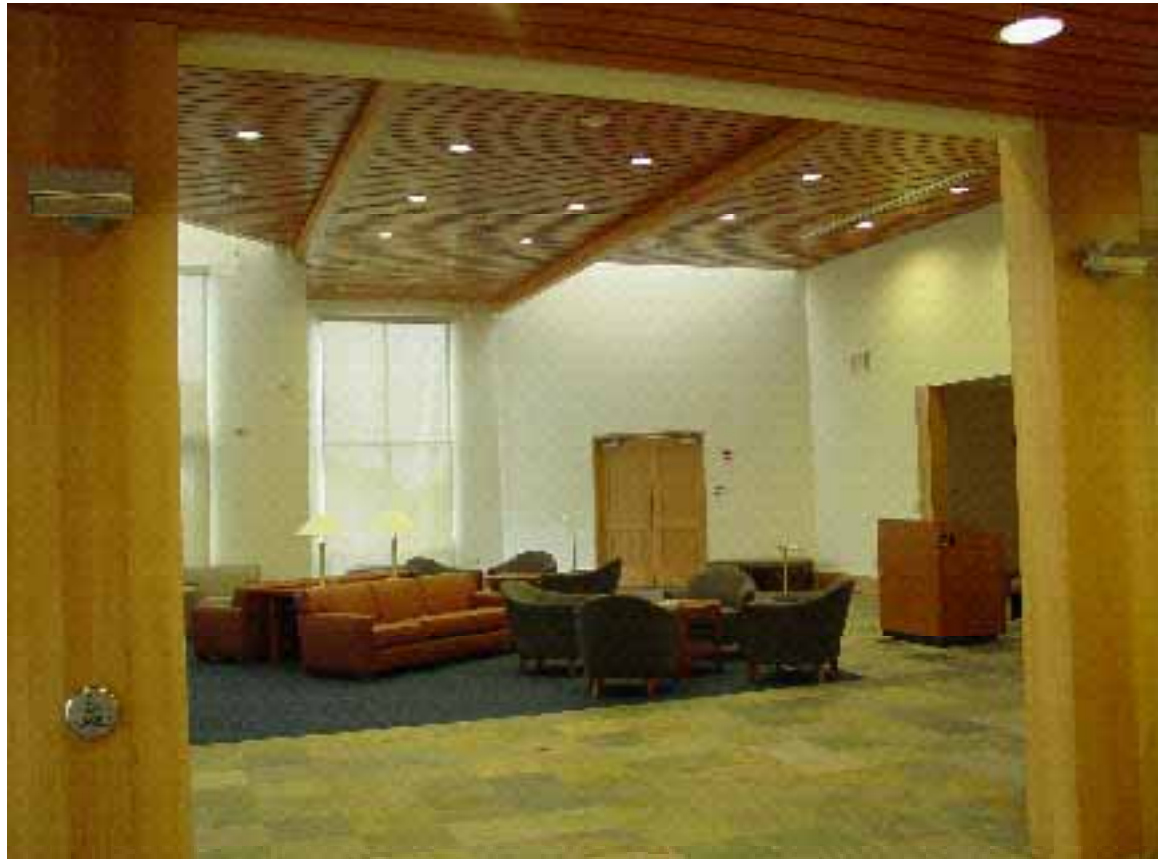
Figure 2.10 Reclaimed wood is reused for a new ceiling at the Cal State University Visitors Center, one of the new institutions at the former Fort Ord.
