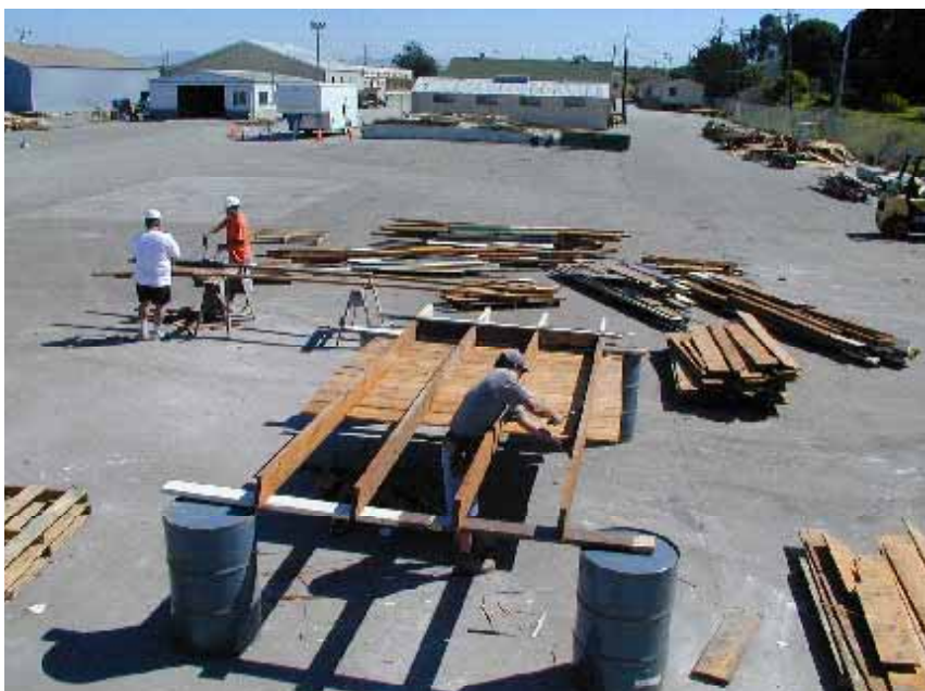
Figure 2.5 Removing sheathing from joists, the work is elevated for convenience
